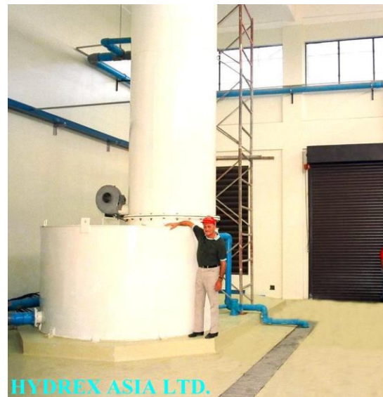
A two train strong acid cation exchanger with degasifier installed in a bottling plant in Calasiao, Philippines to replace an existing lime soda dealkalization / softening system.
