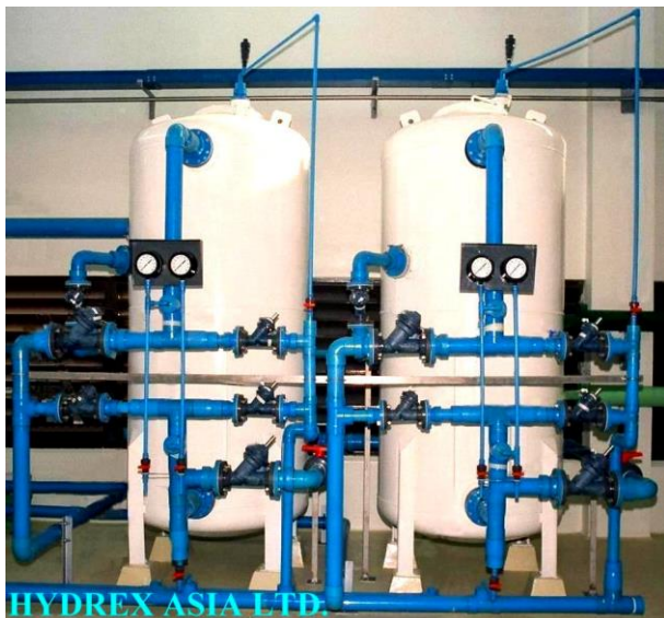
A two train strong acid cation exchanger with degasifier installed in a bottling plant in Calasiao, Philippines to replace an existing lime soda dealkalization / softening system.
