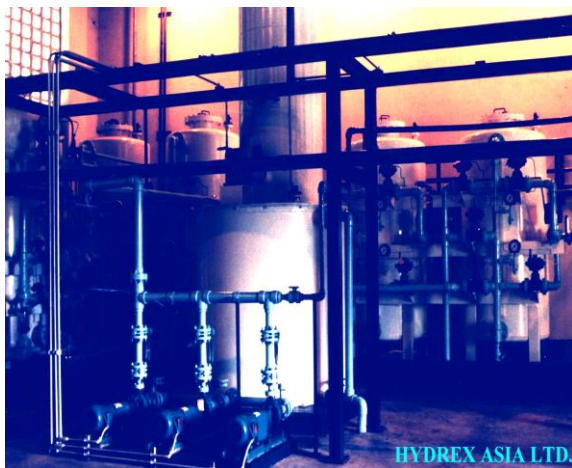
A fully automatic two train 900m 3 /day demin. System is equipped with polishing mixed bed to produce ultra pure water for La Tondena Inc., Philippines.
