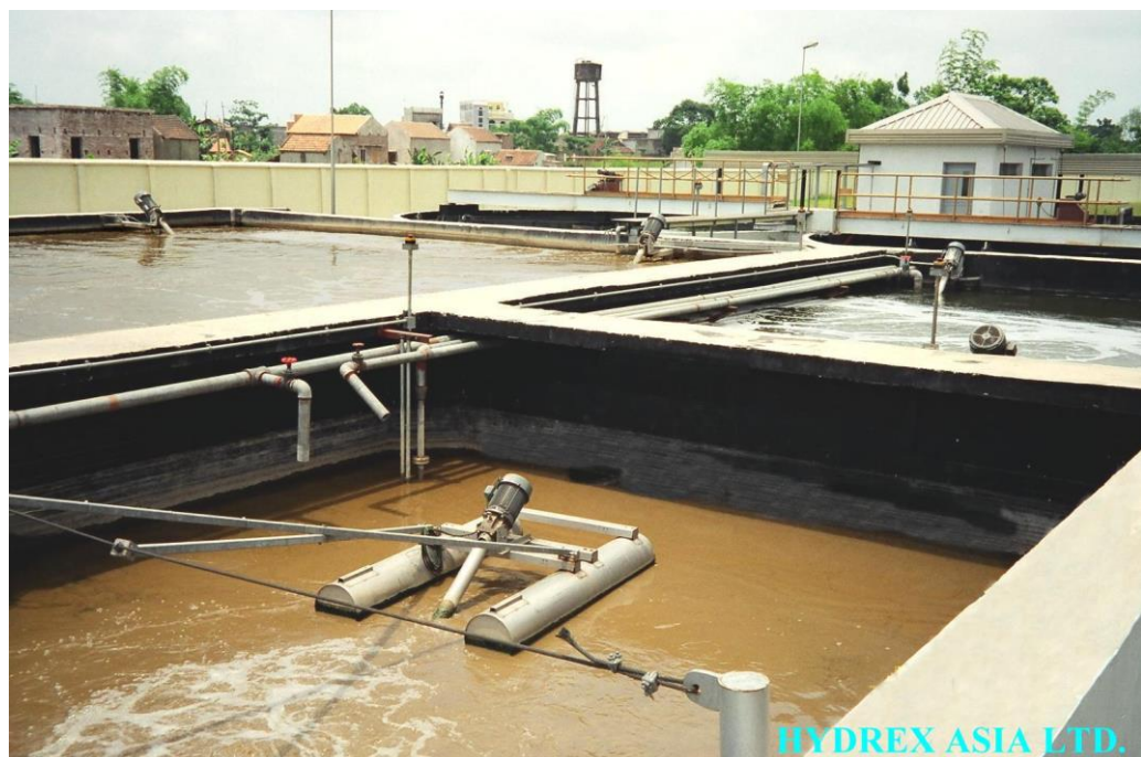
Two-stage Activated Sludge (high rate and nitrification) Wastewater Treatment Plant
