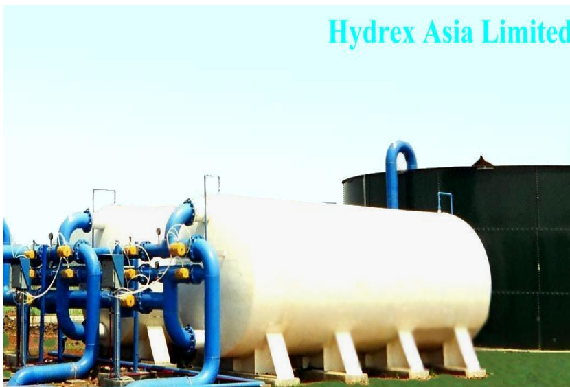
2.4m diameter automatic horizontal filters for an industrial park water supply system.
