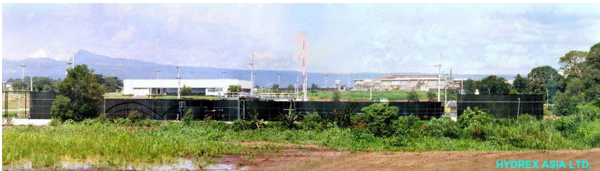
Centralized Wastewater Treatment Plant for Light Industry & Science Park of the Philippines (LISP-I) in Cabuyao, Laguna
