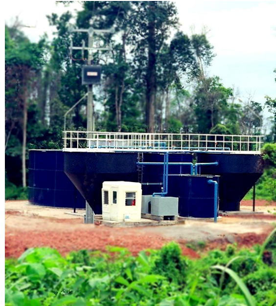
400 cu. m/day sewage treatment plant (Net area 195 sq. m)
