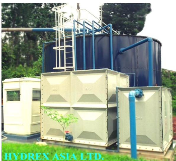
70 cu. m/day sewage treatment plant (Net area 57 sq. m)
