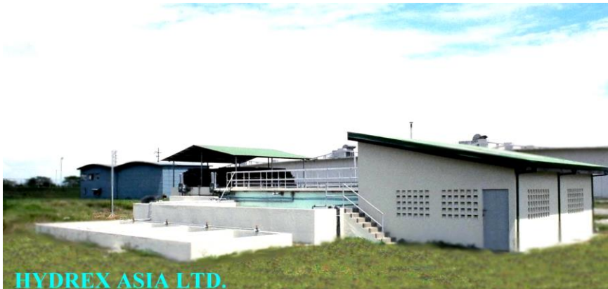
Wastewater Treatment System for Coca Cola's Concentrate Plant in the Philippines
