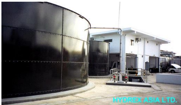
Glass Fused Steel Process Tanks
