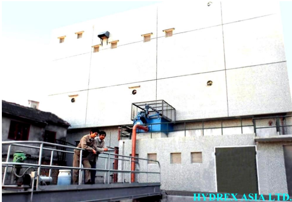
Enclosed Multi-Story Wastewater Treatment plant for Hua Guang Brewery, Shanghai
